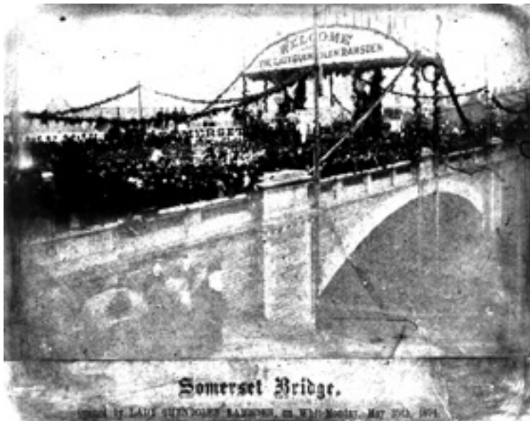
44. Opening of Somerset Bridge by Lady Guendolen Ramsden, 25 May 1874. Kirklees Image Archive
